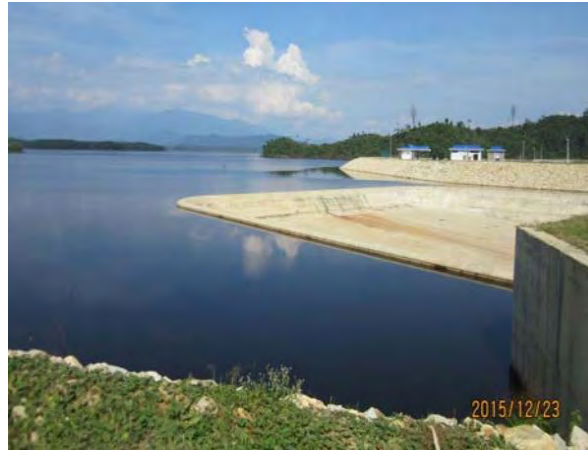
Figure C.12: Ogee Crest Spillway – Kelau Dam (provided by JPS Malaysia)
