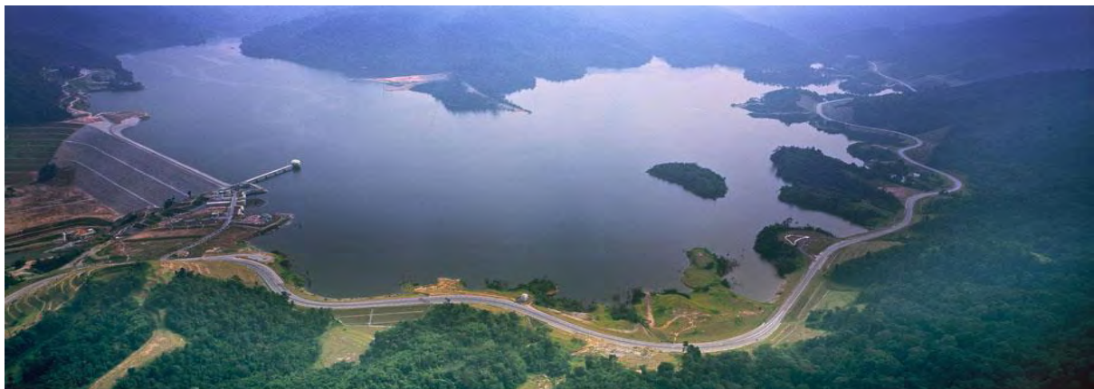
Figure C.4: Clay Core Rockfill Dam – Sungai Selangor Dam (provided by Syarikat Pengeluar Air Sungai Selangor, SPLASH)
