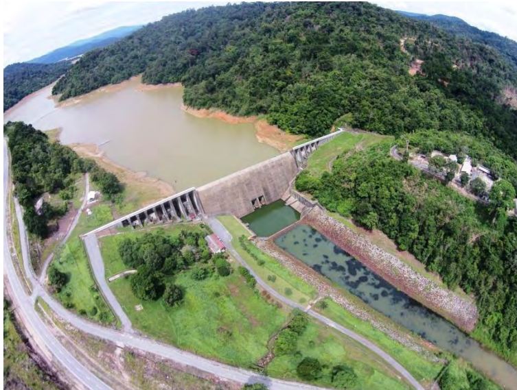
Figure C.8: Concrete Buttress Dam – Muda Dam (provided by Lembaga Kemajuan Pertanian Muda)
