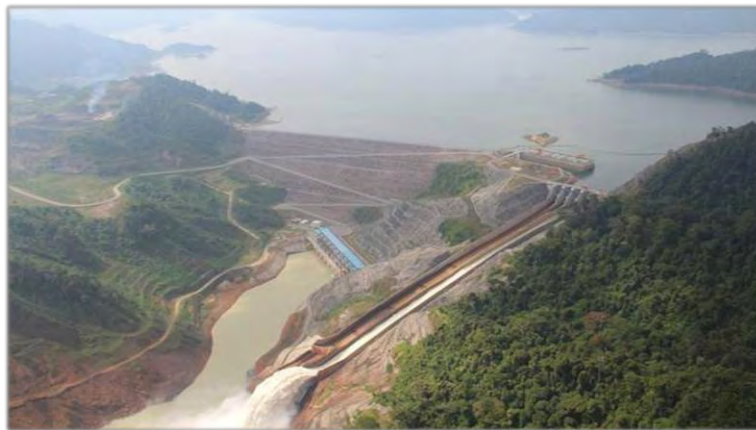
Figure C.3: CFRD – Bakun Dam (provided by Sarawak Hidro Sdn Bhd)
