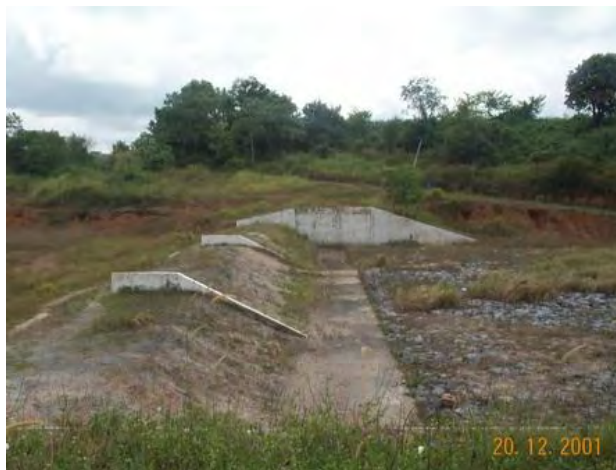
Figure C.15: Auxiliary Spillway – Timah Tasoh Dam (provided by JPS Malaysia)
