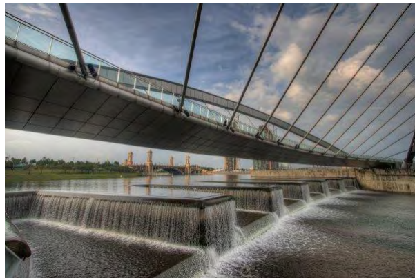
Figure C.13: Labyrinth Spillway – Putrajaya Dam (provided by Perbadanan Putrajaya)
