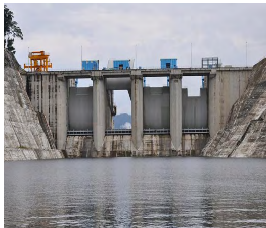
Figure C.9: Crest Mounted Radial Gates – Bakun Dam (provided by Sarawak Hidro Sdn. Bhd.)
